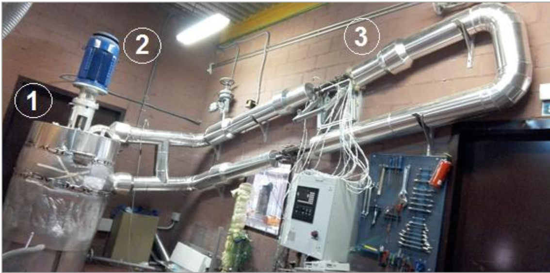
Figure 17: Circulation of the molten salts experiment installation.
