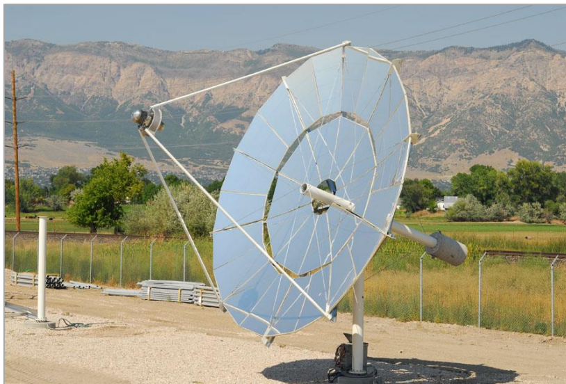
Figure 12: Parabolic Dish at Maricopa power plant.
