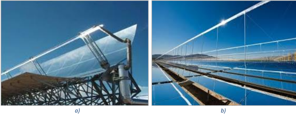
Figure 11: a) Parabolic Trough. b) Fresnel.
