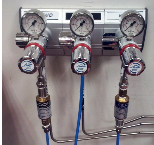
Figure 4.26: Gas flow regulation system. From left to right: propane, nitrogen and oxygen lines
