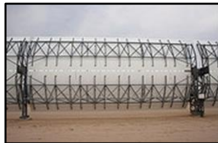
Figura 44. Estructura del colector LS-3 (National Renewable Energy Laboratory (NREL)).
