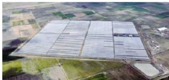
Lebrija, Spain: The Andalusian concentrated solar power (CSP) plant is one of the more than 40 CSP projects worldwide, where a SST-700 reheat steam turbine was chosen.
