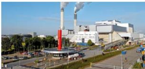
Amsterdam, Netherlands: AEB's waste fired power plant uses a 74 MW(e) extraction condensing turbine in reheat configuration.
