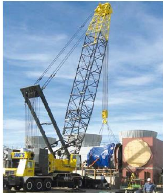
Installing the SST-700 LP turbine on the concentrated solar power plant in Boulder City, Nevada, USA.
