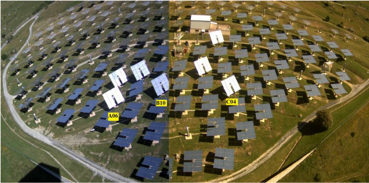
Figure 3.4: Photograph of THEMIS heliostat field from the receiver. Selected heliostats are marked.
