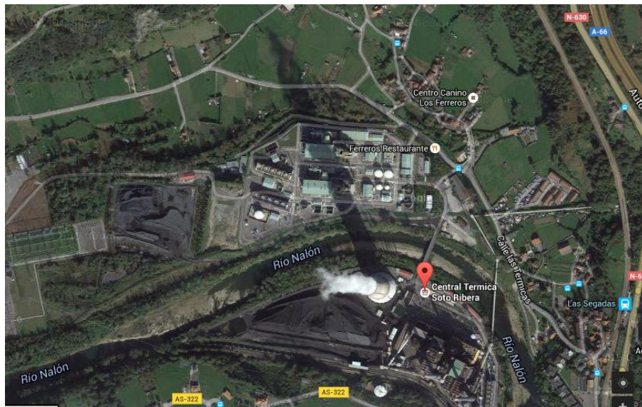
Figure 30. Soto de Ribera thermal power plant seen from above.
