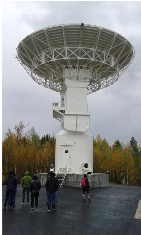
FIGURE 18.3. Radio telescope of the Finnish Geospatial Research Institute (FGI) at the Metsähovi research station, used for geodetic very long baseline interferometric (VLBI) observations. The telescope, aperture 13.2 m, belongs to the international VLBI Global Observing System (VGOS).
