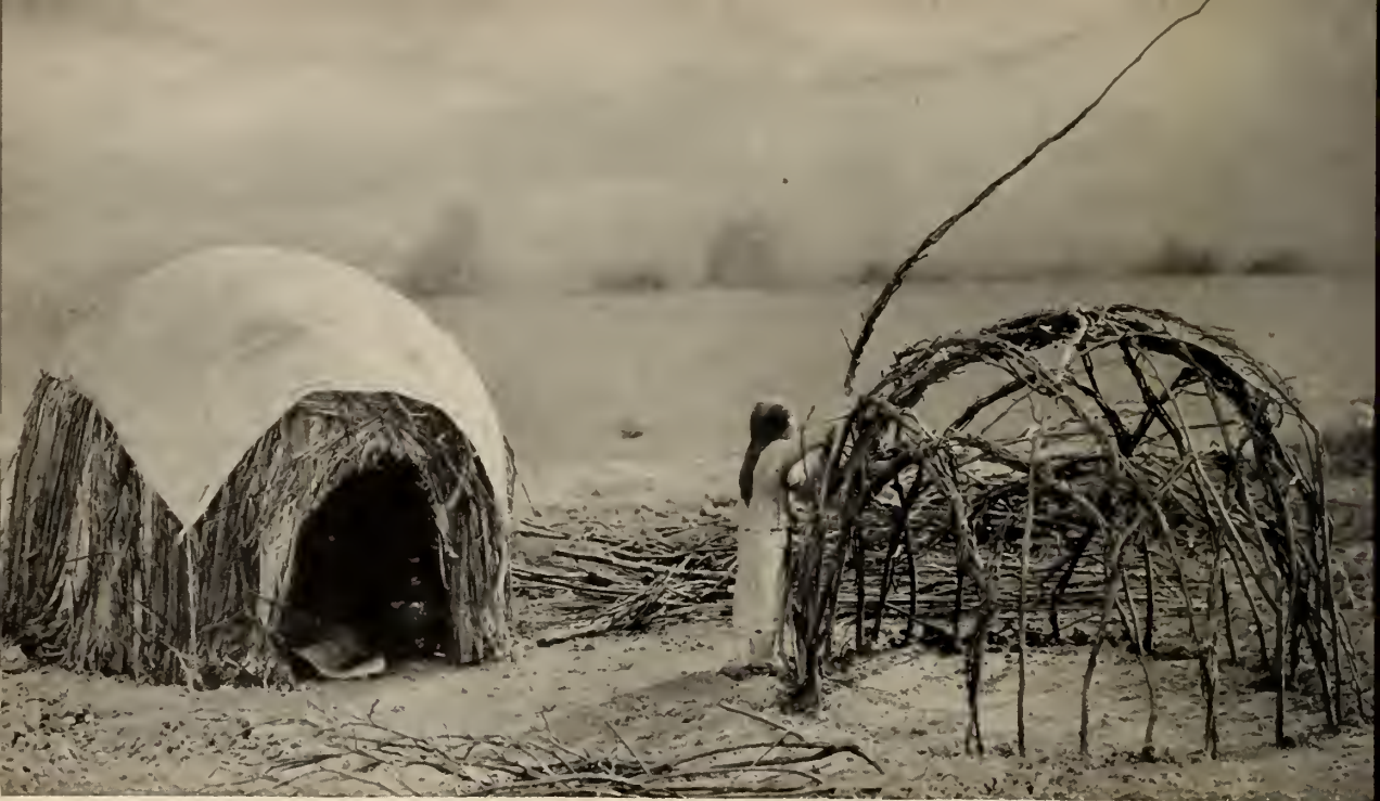
(Above) APACHE WOMAN BUILDING FRAMEWORK OF A HOUSE to be covered with thatch and rushes
