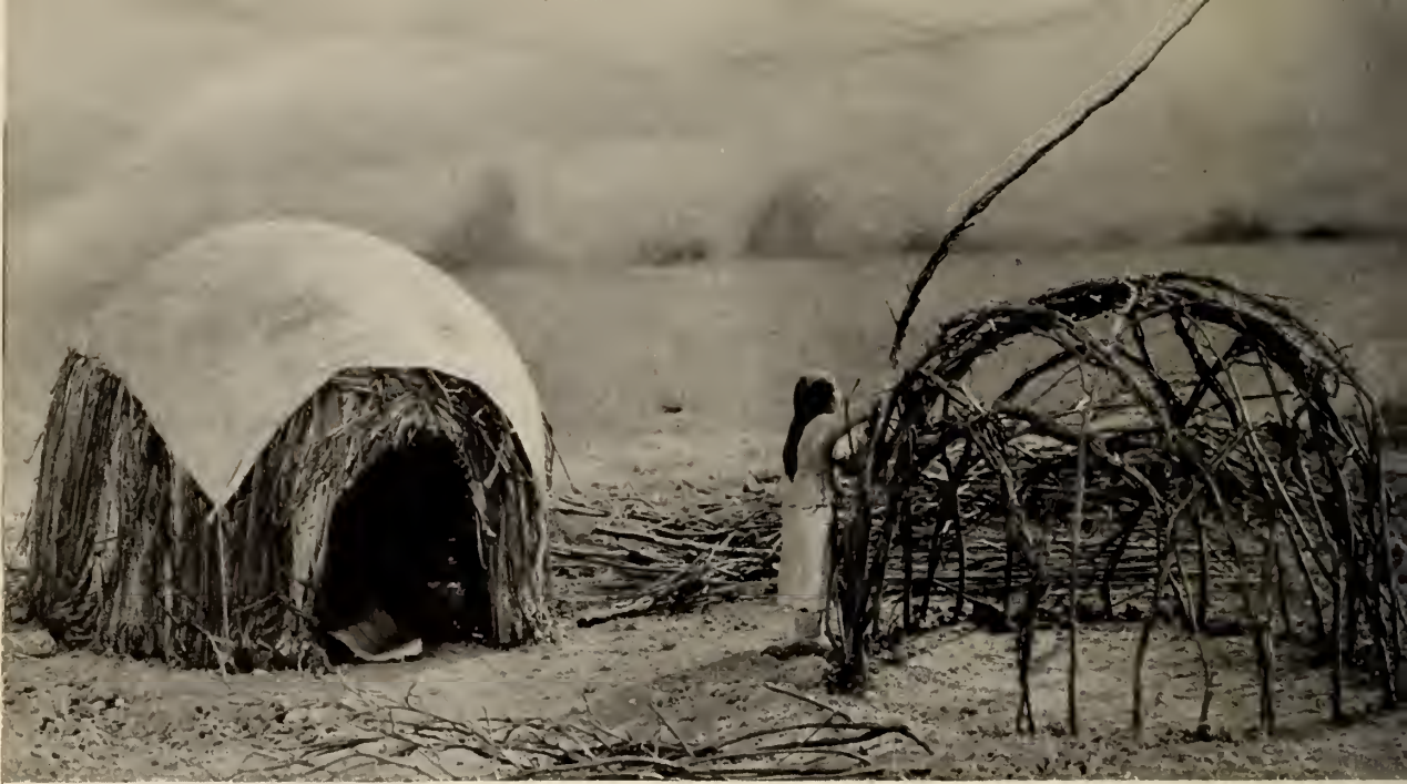
(Above) APACHE WOMAN BUILDING FRAMEWORK OF A HOUSE to be covered with thatch and rushes
