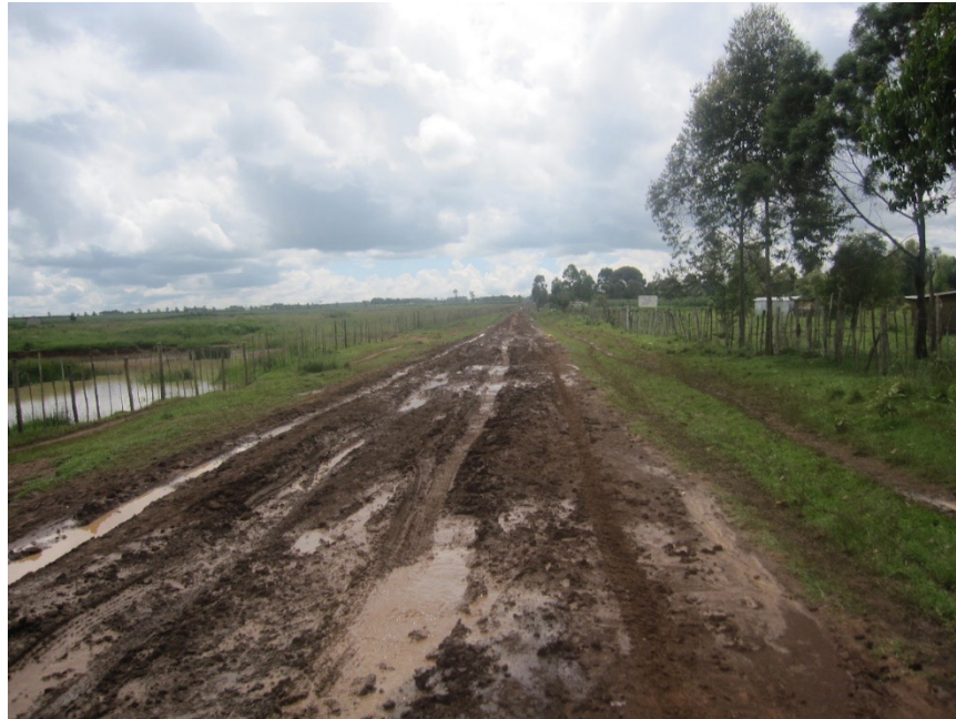
Photo 1: a rural road outside of Eldoret which becomes unusable for ordinary passenger cars and pick-up trucks after a heavy rain.
