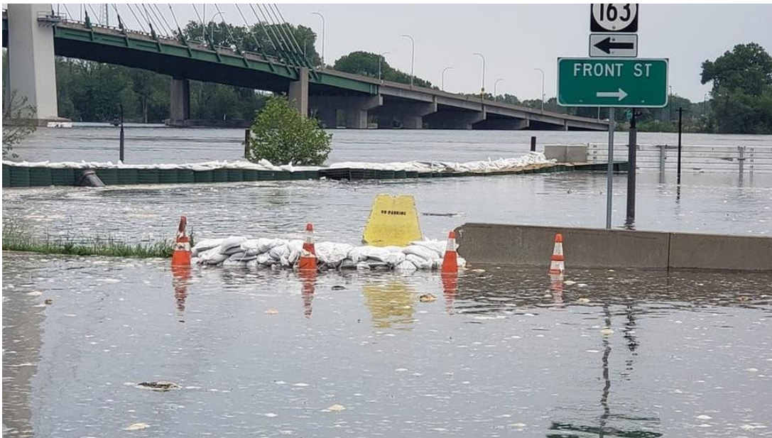
Figure 1: Emergency Flood Barriers 1
