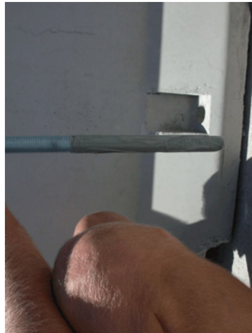
Figure 11. Barrier Tie-Down Installation
