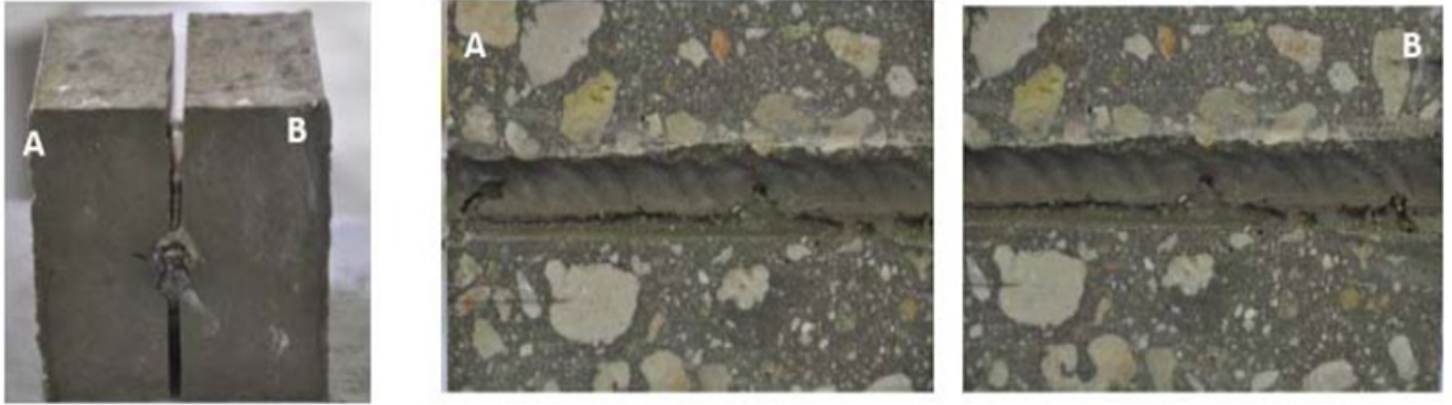
Fig. 3: Bisecting of the area around the reinforcement
