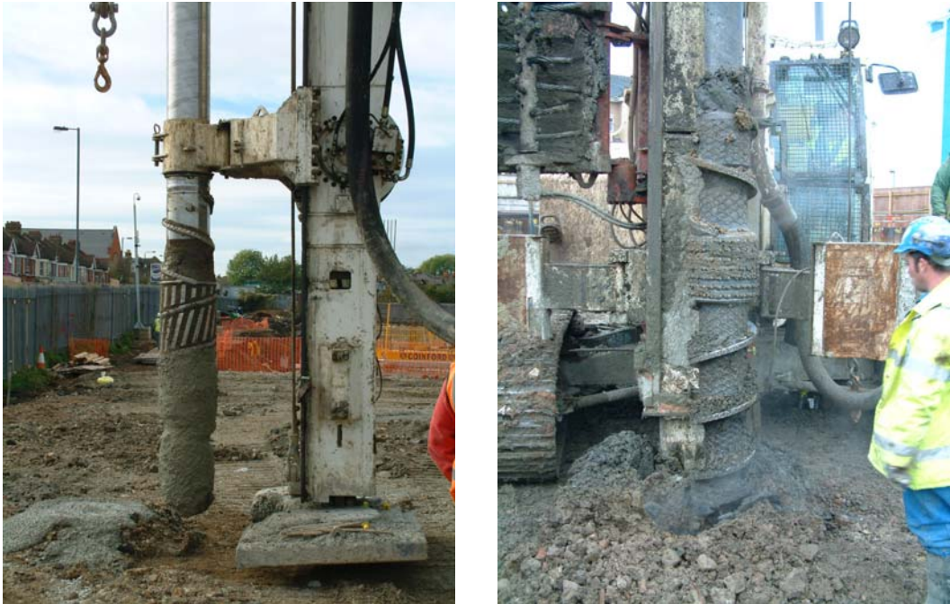
Figure 2.12. Third generation BD pile augers in use.
