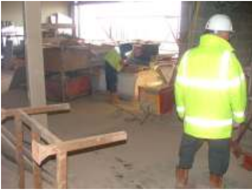
Figure 4.1 Congested work site
