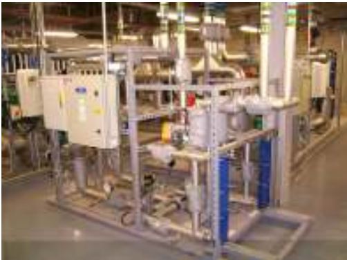
Figure 4.40 Plantroom module, type A materials (MTO)
