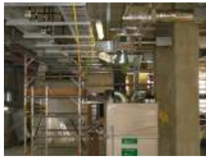
Figure 6 Various trades in same workplace, materials in each trades way
