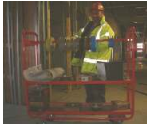
Figure 8 Mobile cable dispensing and component trolley with simple manual replenishment
