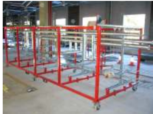
Figure 4.32 ATIF module ready for installation, type A materials (MTO)
