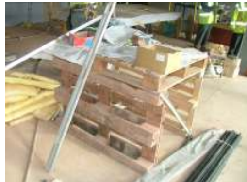
Figure 4.6 Congested and improvised workplace
