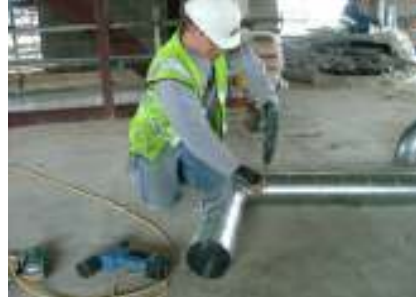
Figure 2 Working on the floor
