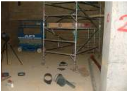
Figure 5 Unplanned workplace, conventional scaffold
