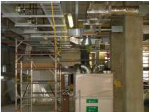
Figure 4.3 Various trades in the same workplace
