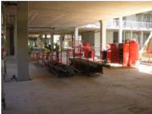
Figure 4.31 Mobile work cell for drainage crews in their own clear space
