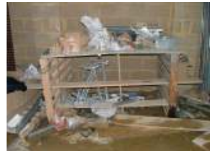
Figure 4 Improvised workbench and random storage of components
