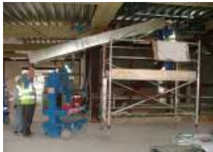
Figure 3 Conventional scaffolding and manual handling
