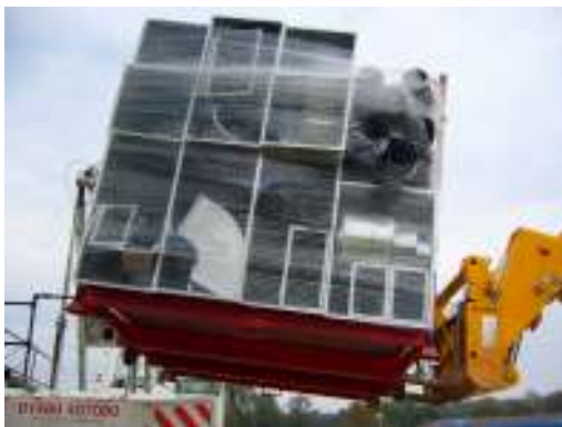
Figure 2 Kit of parts for ventilation system on mobile stillage
