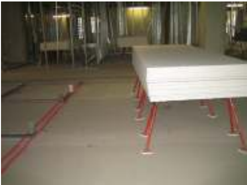
Figure 4.38 Ergonomic materials handling equipment for dry-lining boards
