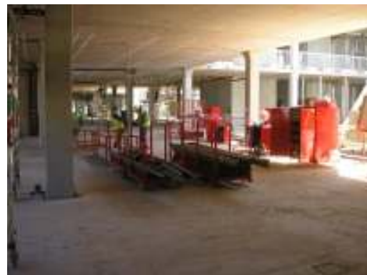
Figure 3 Mobile work cell – drainage crew
