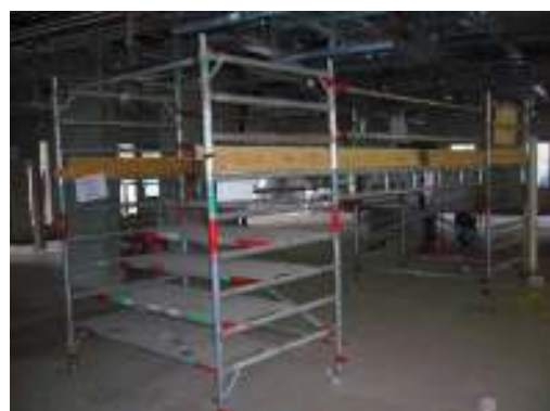
Figure 4.36 Ergonomic access equipment, walk-up mobile scaffold
