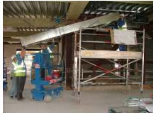
Figure 4.2 Manual handling onto a scaffold
