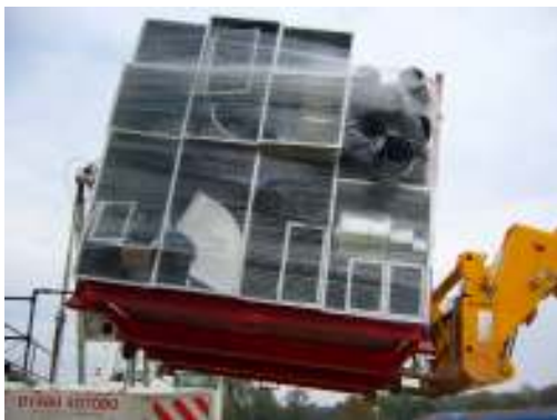
Figure 4.33 Kit of parts for ventilation systems on mobile carrier, type B materials (MTO); inbound logistics
