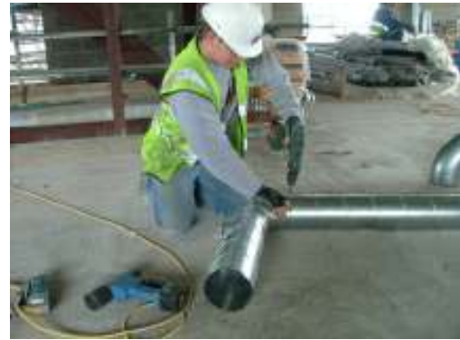
Figure 4.4 Working on the floor
