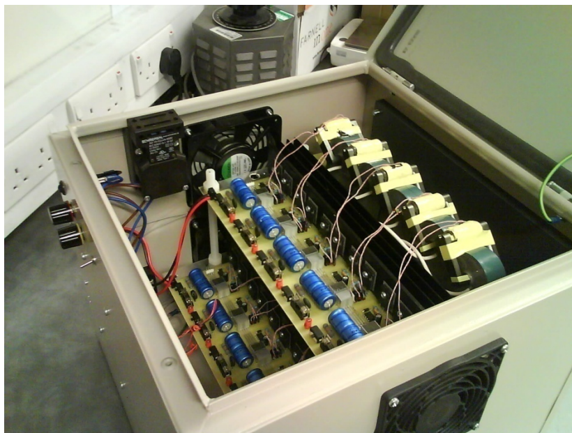
Figure 3.22 Photograph of completed power supply
