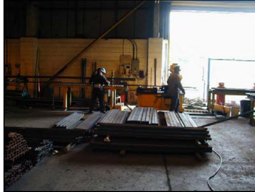
Figure 5.14 Modular building manufacture; welding fumes from channels
