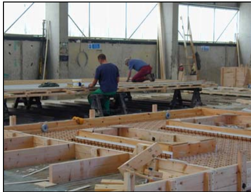
Figure 5.6 Offsite manufacture of panel moulds; trunk movement
