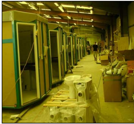
Figure 5.4 Offsite manufacture of washroom toilet pod
