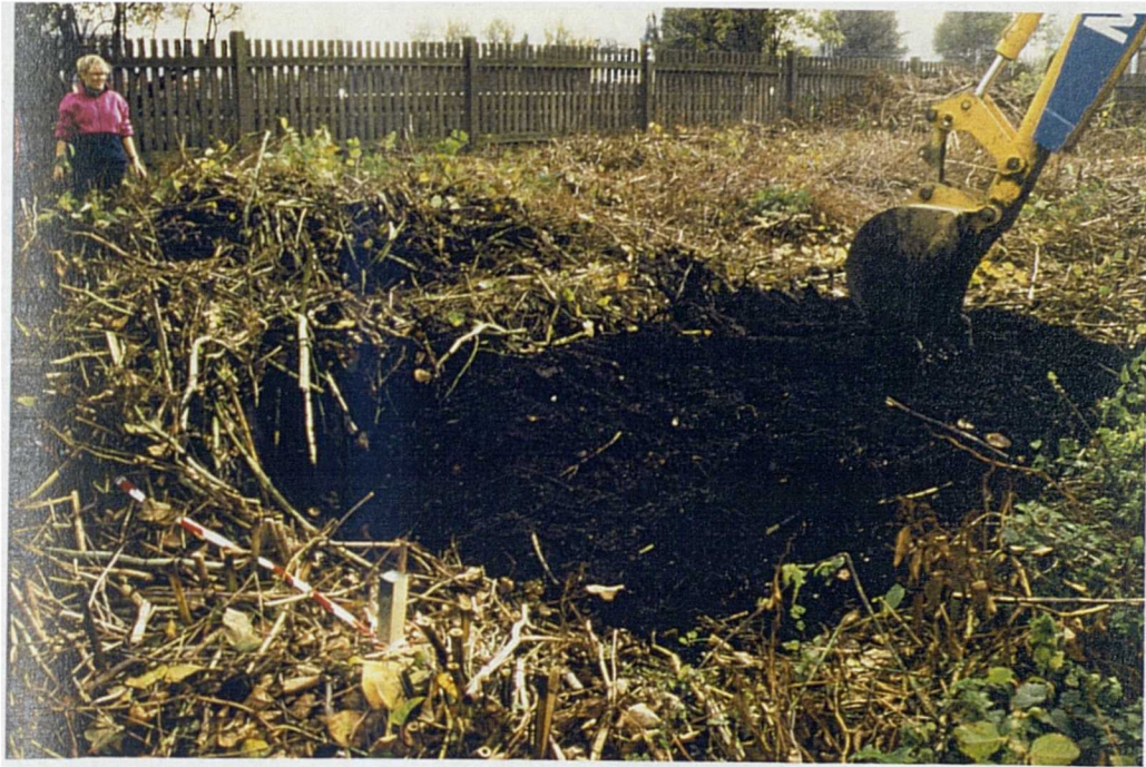
Figure 5.3 Photograph of trial site during site preparation in October 1993 showing digging procedure on plots 2 and 3. Note extensive cover of F. japonica material.
