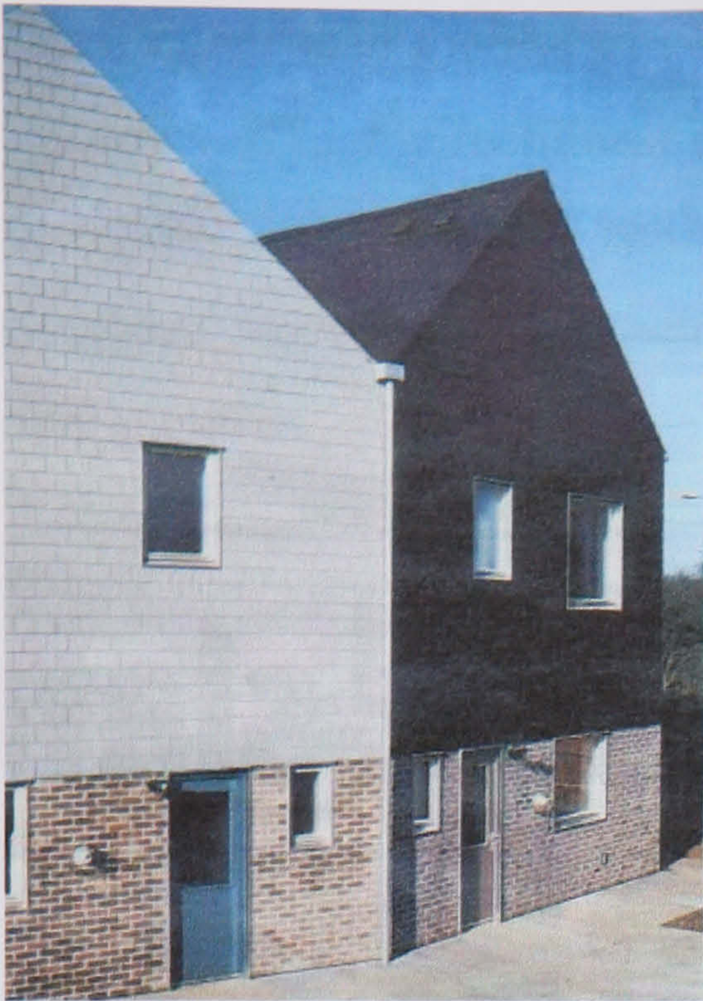
Figure 8.7 Semi-detached house Stevenage, UK (Architects: Sergison Bates)
