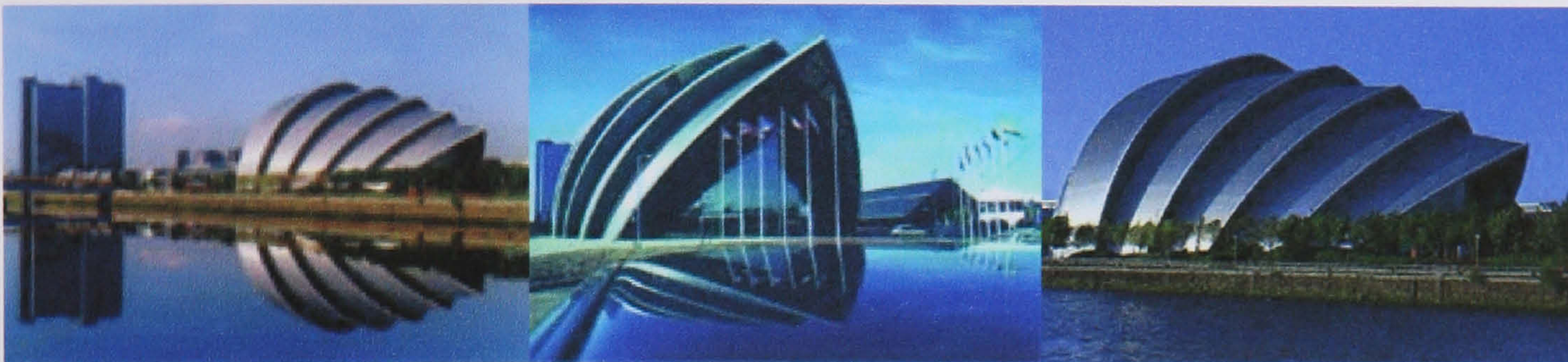
Figure 8.6 The Scottish Exhibition and Conference Centre (SECC) in Glasgow (Architects: Foster and Partners)
