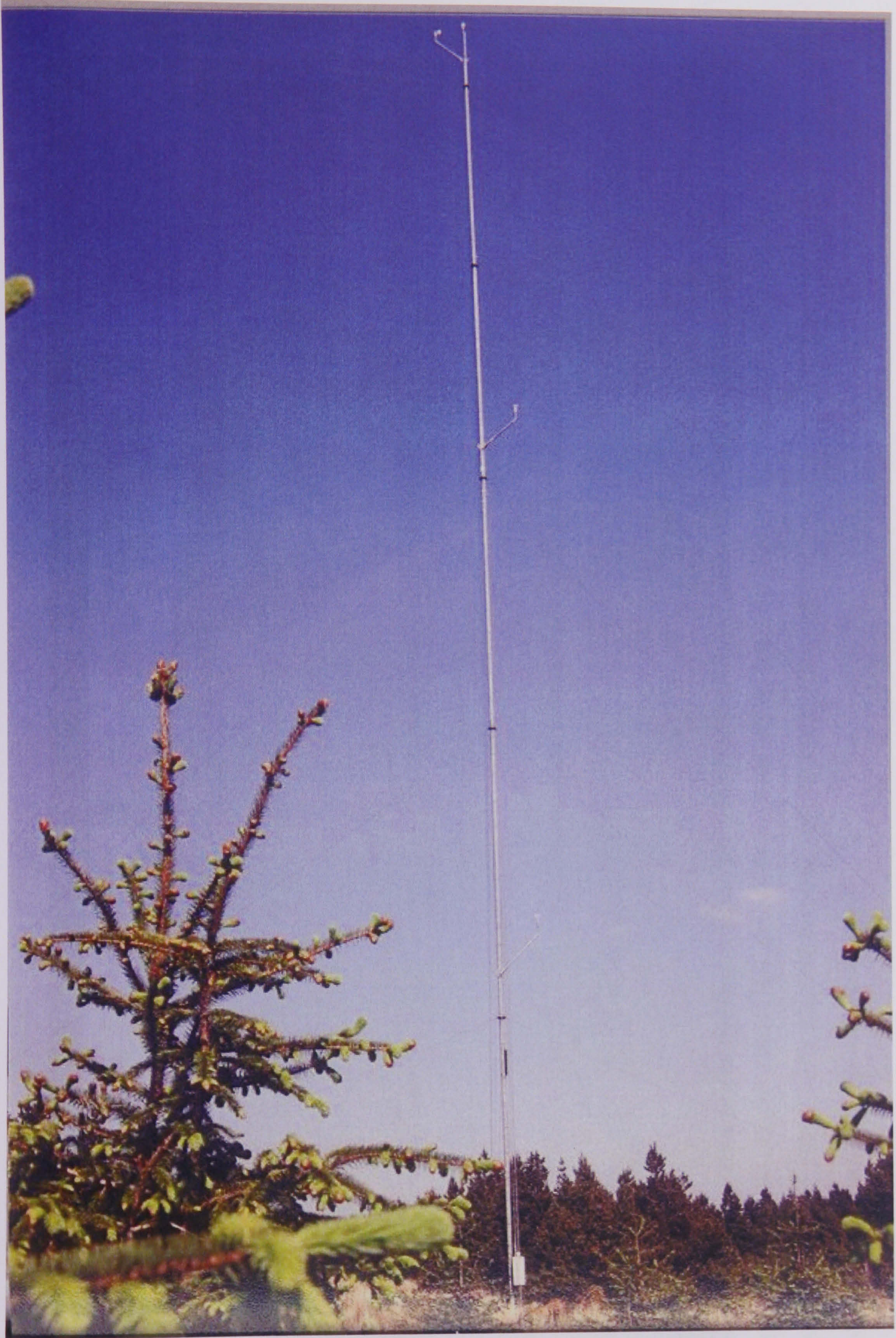
Figure 7.5 - View of anemometer mast
