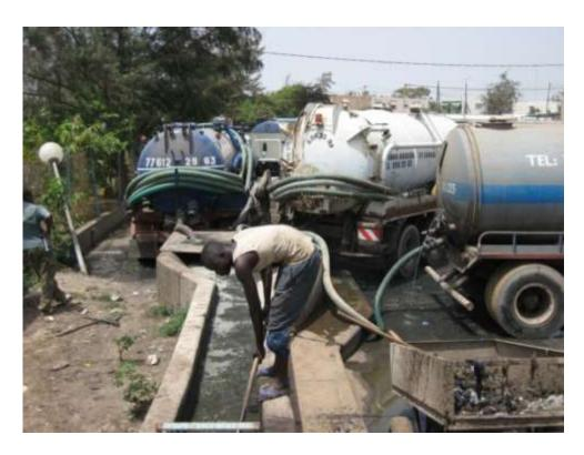
Figure 10-20: FS treatment centre Cambarène Dakar, worker manually removing foreign material from grate (taken by author 2008 Dakar)
