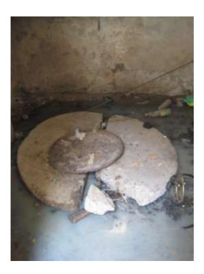
Figure 10-12: Flooded septic tank Pikine Irrégulier Sud (taken by author 2008)<sup>55</sup>.
