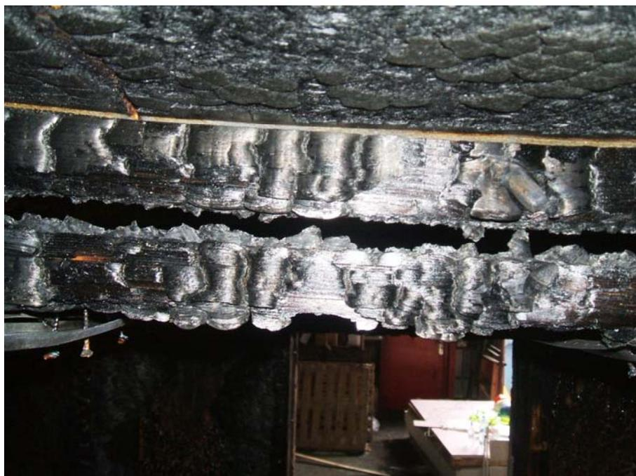
**Figure 4.13**      **Damage to engineered floor systems (F2-EPS30)**
