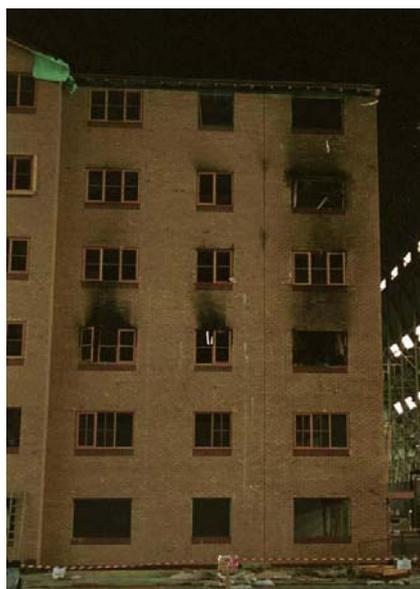
**Figure 2.2** The TF2000 building post fire test
