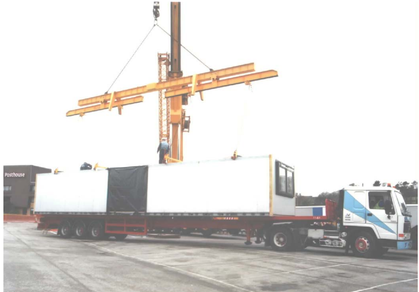
Figure 4 Modular building - Site delivery of steel-framed, double hotel bedroom unit Courtesy of Yorkon Ltd.
