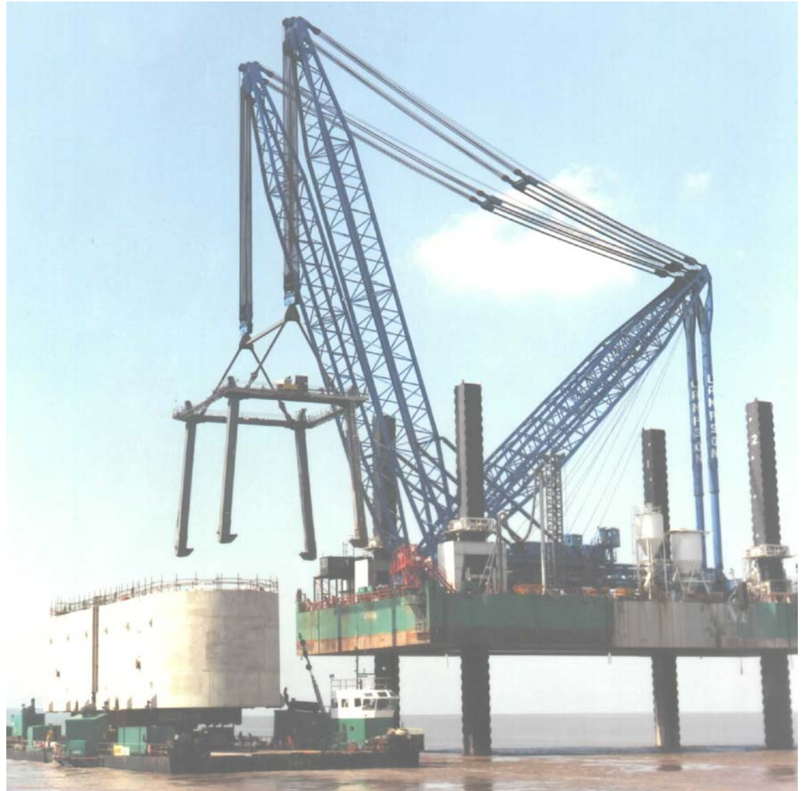
Figure 9 Non-volumetric pre-assembly (complex) - Installation of precast concrete bridge caissons Courtesy of Laing
