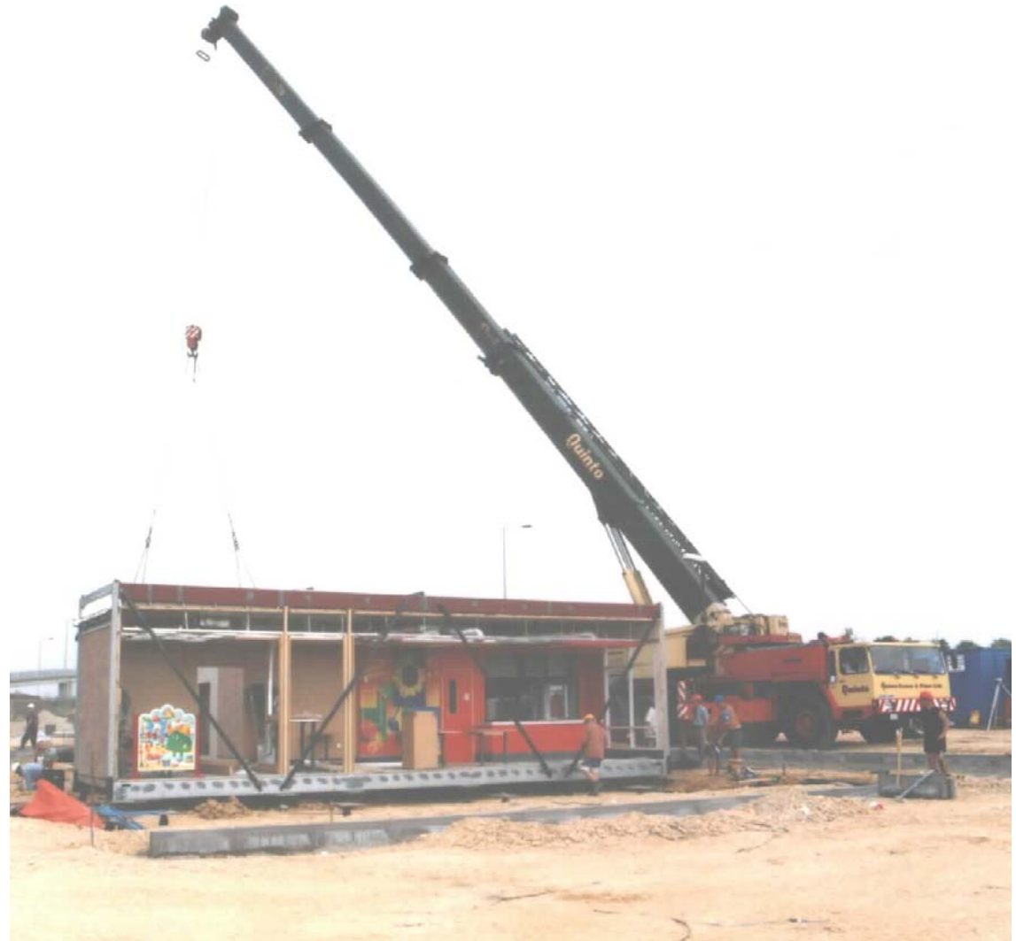
Figure 3 Modular building - Installation of steel-framed unit for McDonald's Restaurants Courtesy of Yorkon Ltd.
