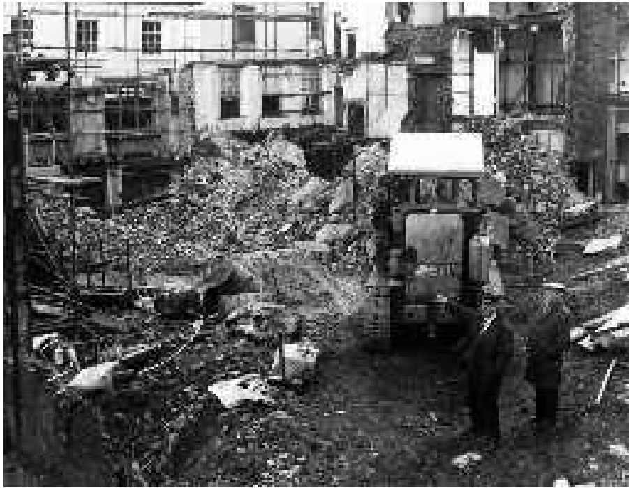
Figure 1.2: Typical 1970's House Demolition. Durham City, Silver Street demolition. ( www.durham.gov.uk )
