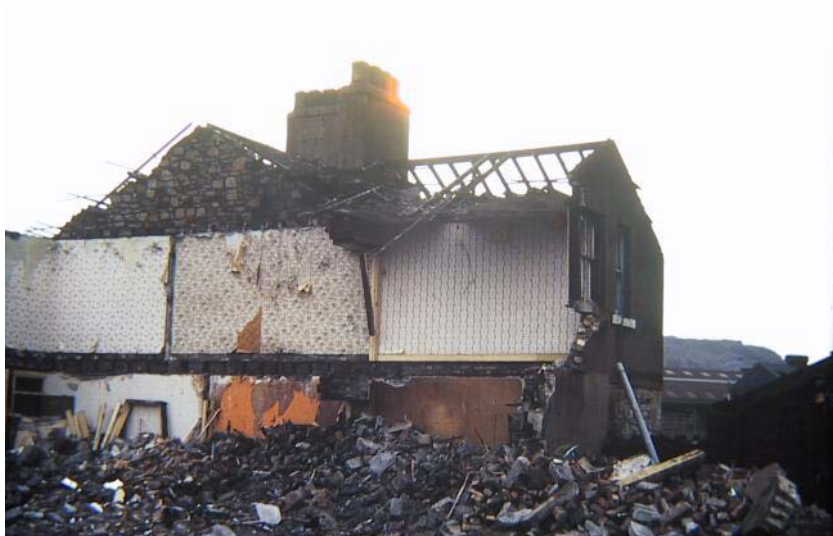
Figure 1.1: Typical 1970's House Demolition Behind Southy Street, Workington. ( www.users.globalnet.co.uk )
