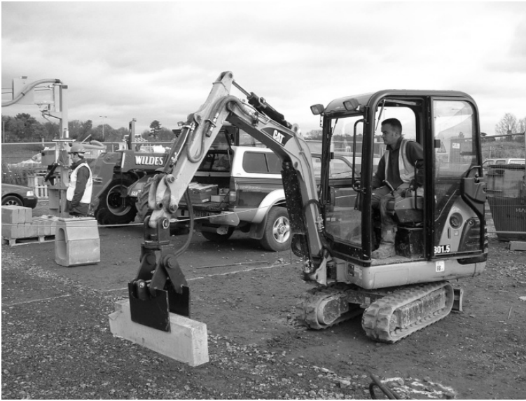
Figure 12 Hydraulic clamp kerb lifter
