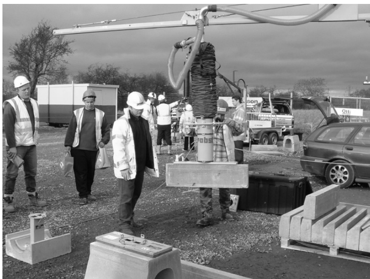
Figure 11 Probst Vacuum lifter with extended tube
