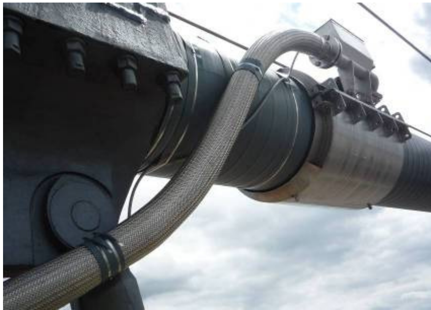
Figure 13: Finished injection sleeve
