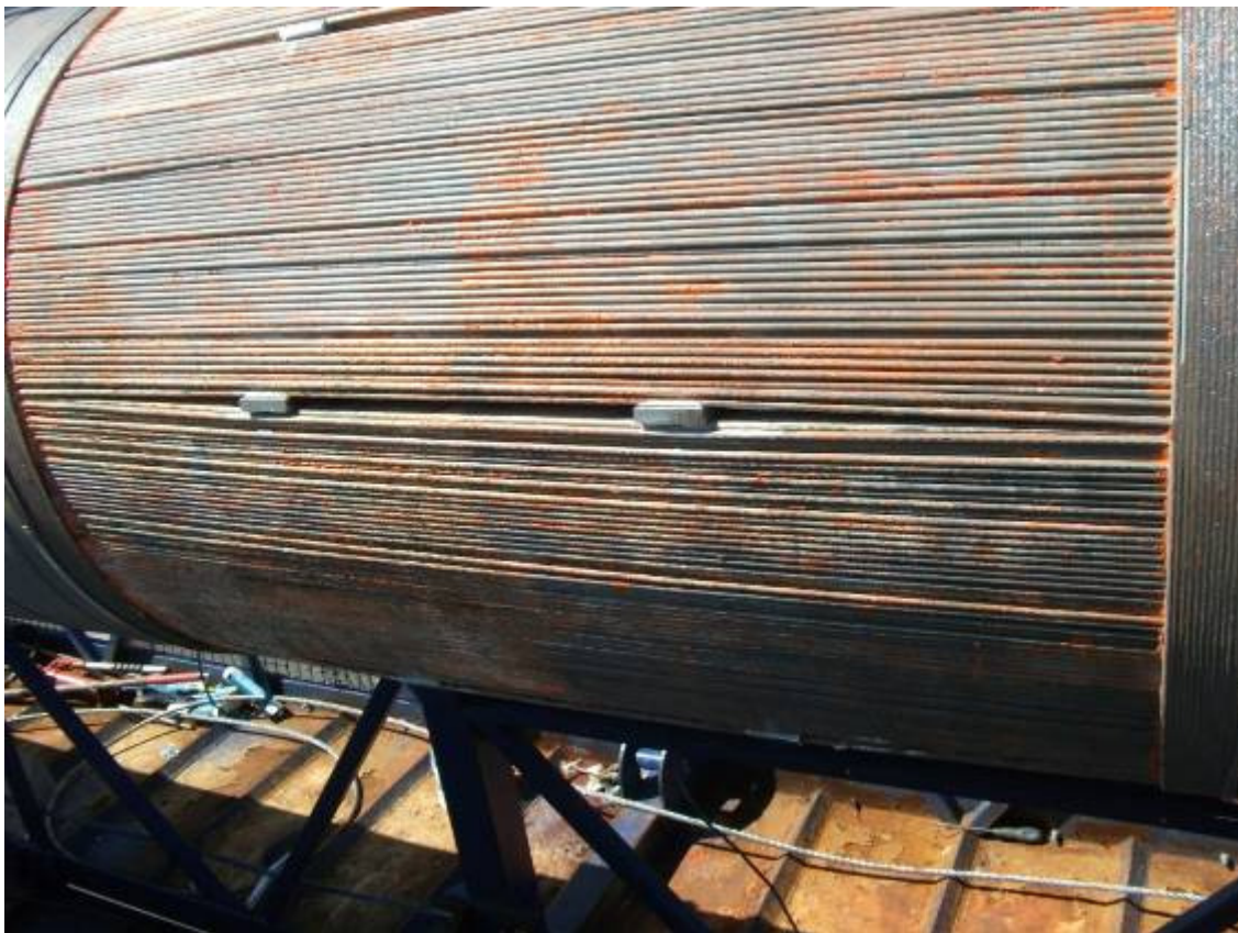
Figure 8: Unwrapped main cable
