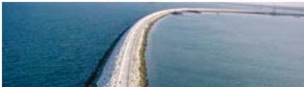
Environmental protection: precast concrete is widely used to protect our coastline
