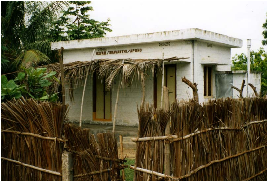
Figure 4: More recent type of ‘cyclone resistant house’ with improvised veranda, built after 2003 (East Godavari, Andhra Pradesh).
