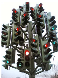
Signalized intersection: traffic control with traffic lights
