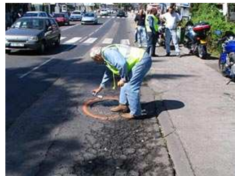
Figure 100: Illustration of road surface defects.
