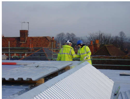
Figure 2 fieldwork in progress
