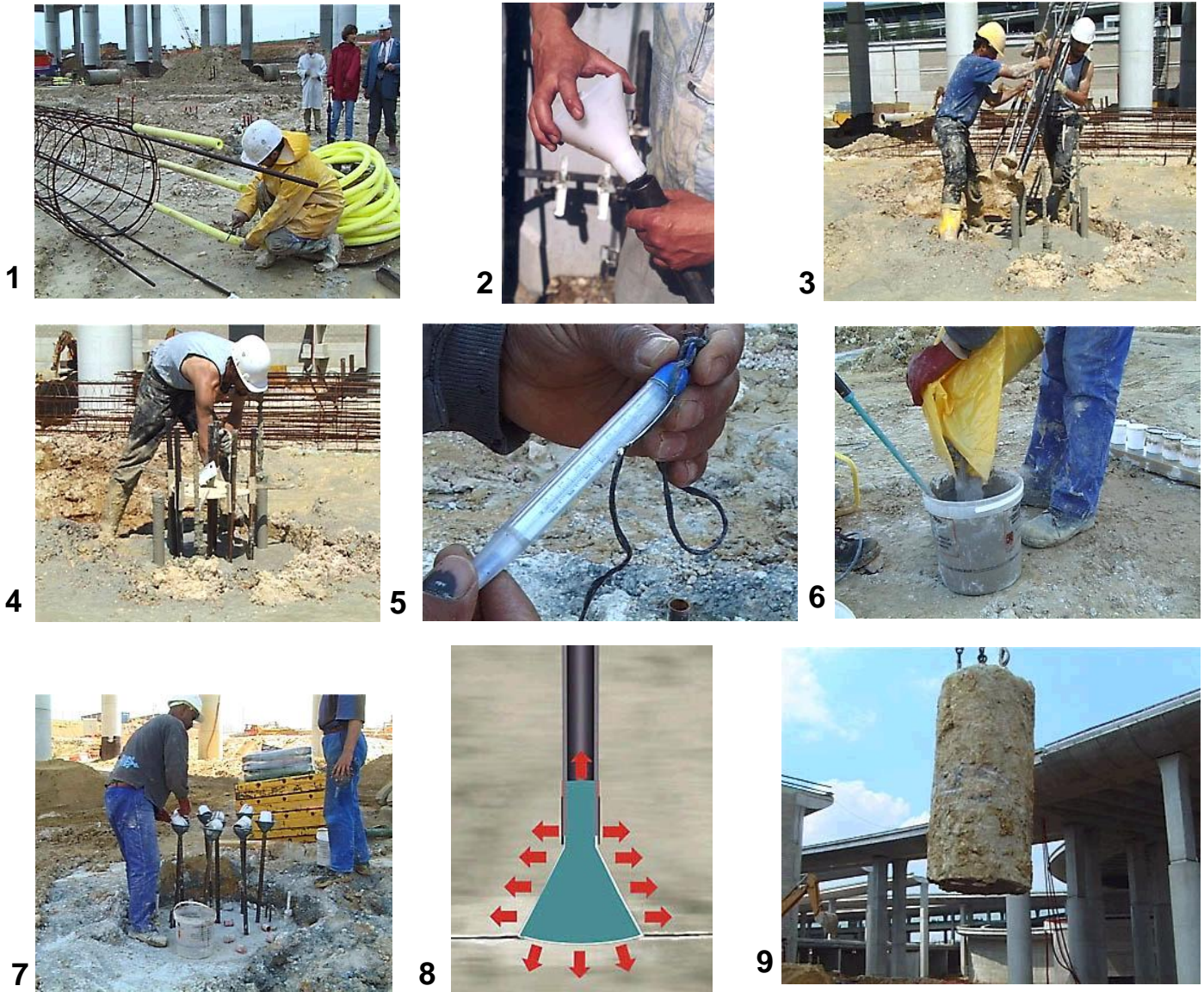
Figure 7 - Recepieux chemical pile breaking method ( http://www.recepieux.com )
