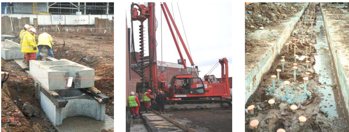
Figure 5 – Cementation sacrificial guide wall (courtesy Cementation)
