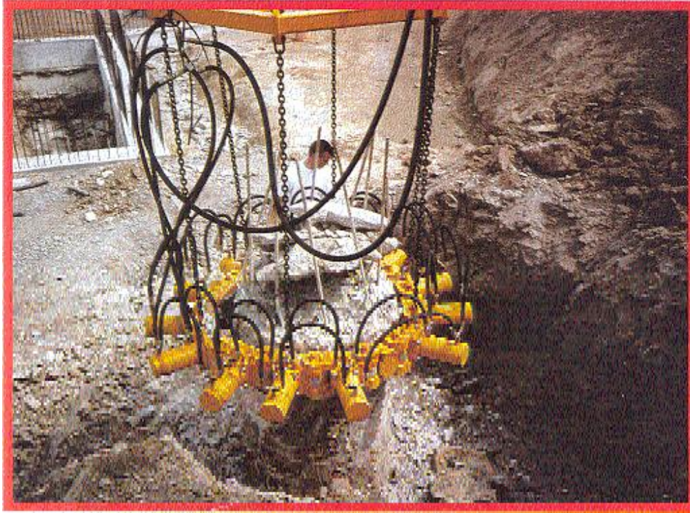
Figure 8 Taets Hydraulic Pile Breaker
