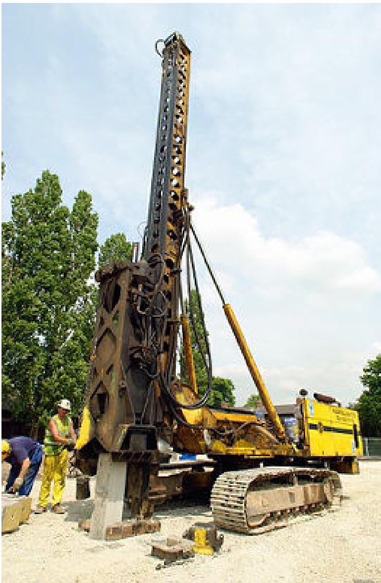
Figure 4 Precast concrete piles (Courtesy Roger Bullivant)
