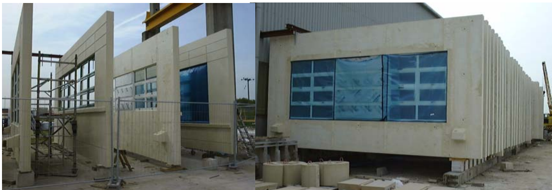
Figure 3 Factory glazing of precast panels at ground level
