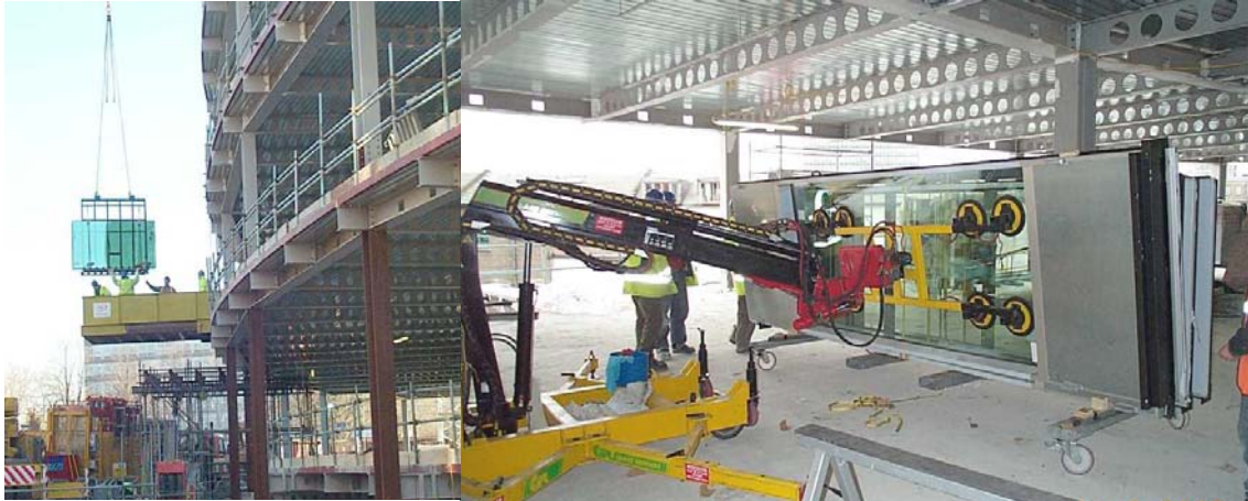
Figure 4 Delivery and distribution of units (Courtesy Bovis-Lendlease)
