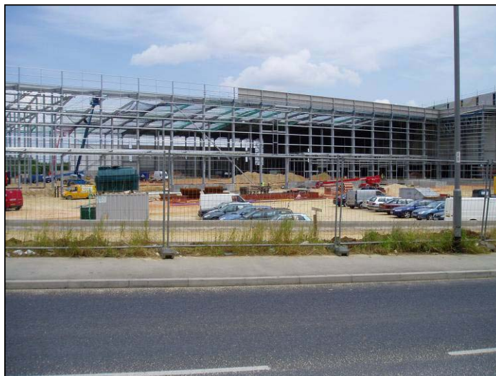
Figure 5. Steel Construction site
