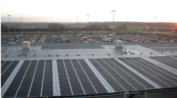
Figure 2: Triple junction amorphous modules on the site in Northern Germany.
