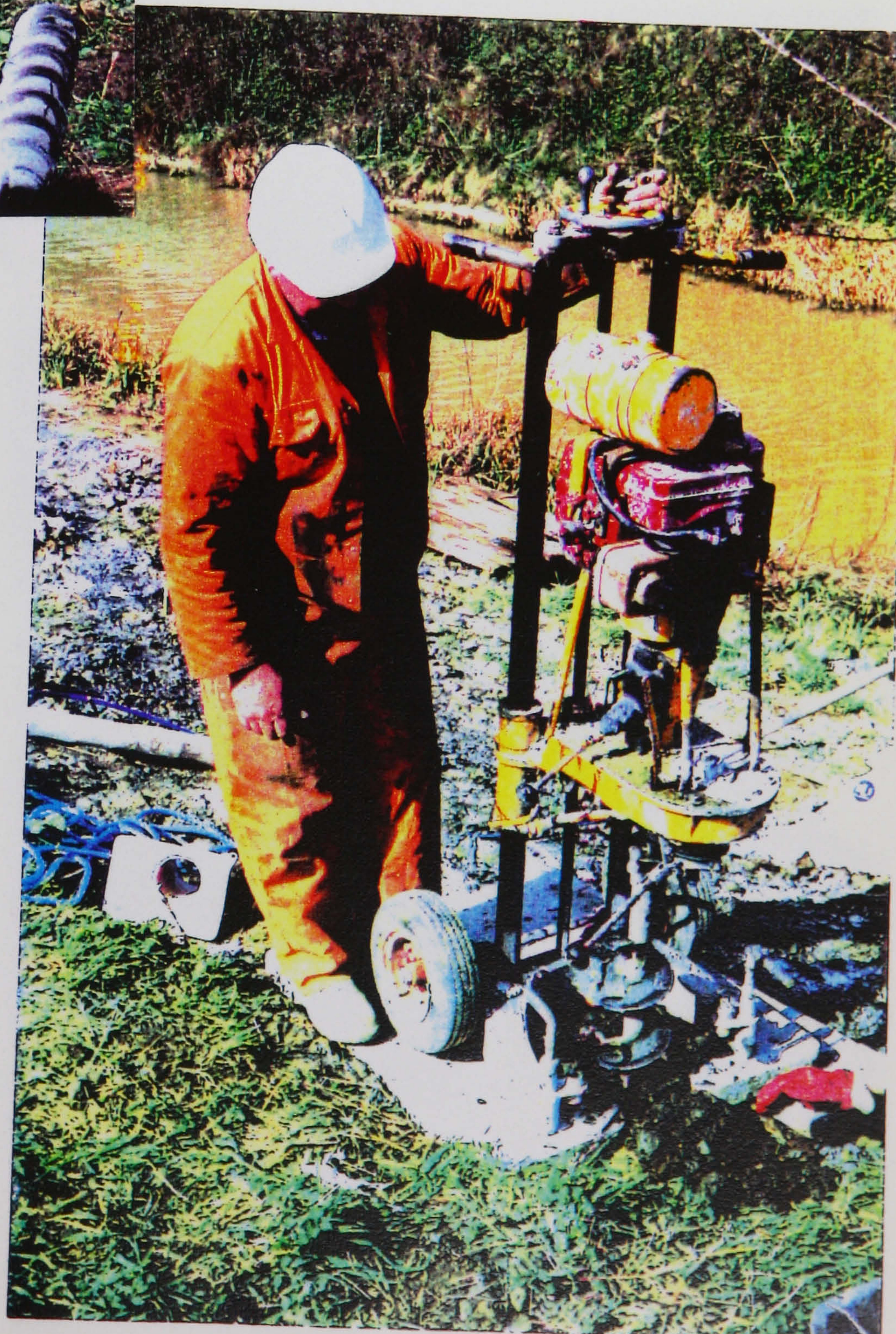
Figure 8.12 Pile installation using a 'Minute-Man' rig
