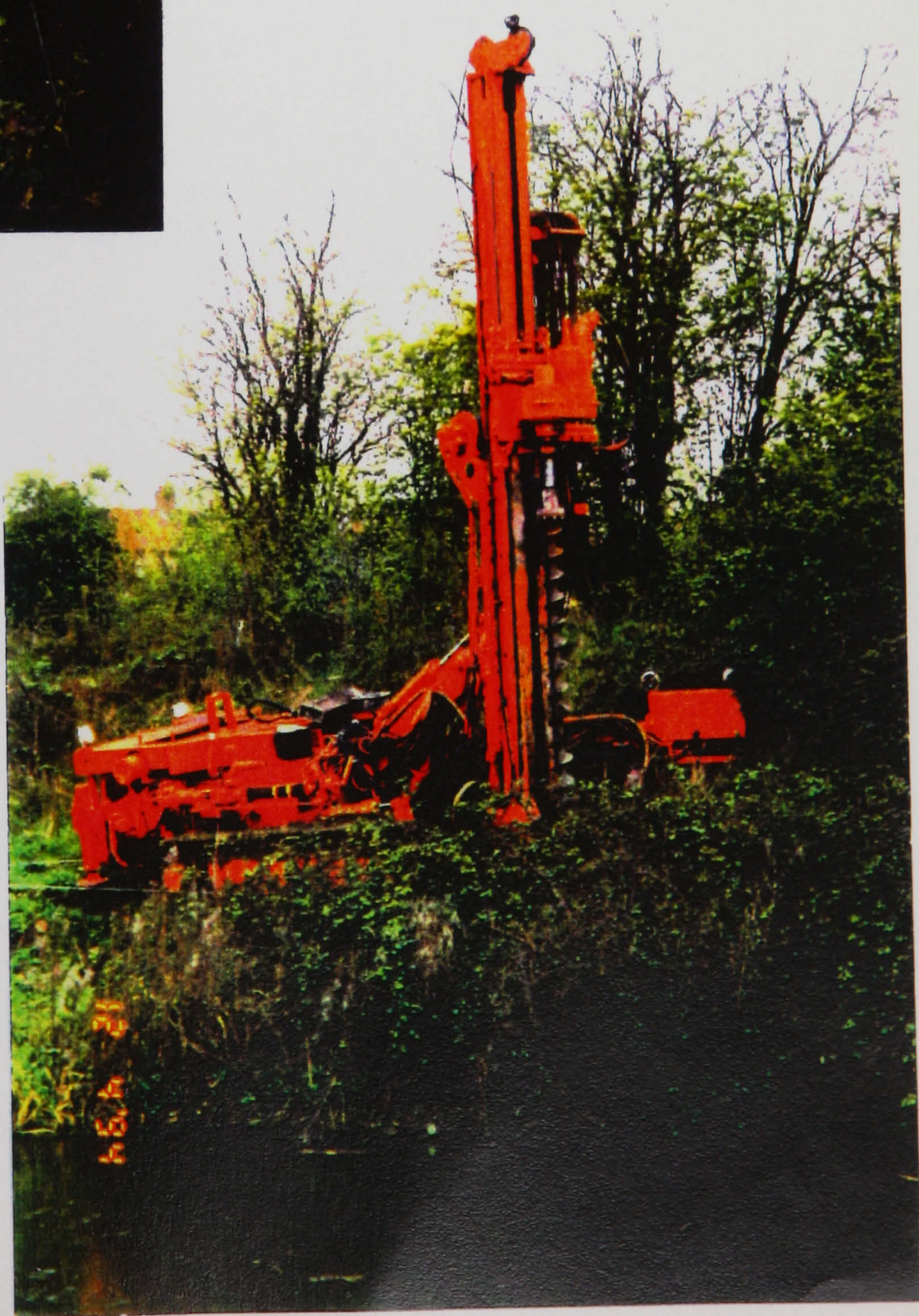
Figure 8.24 Pile installation at Iver
