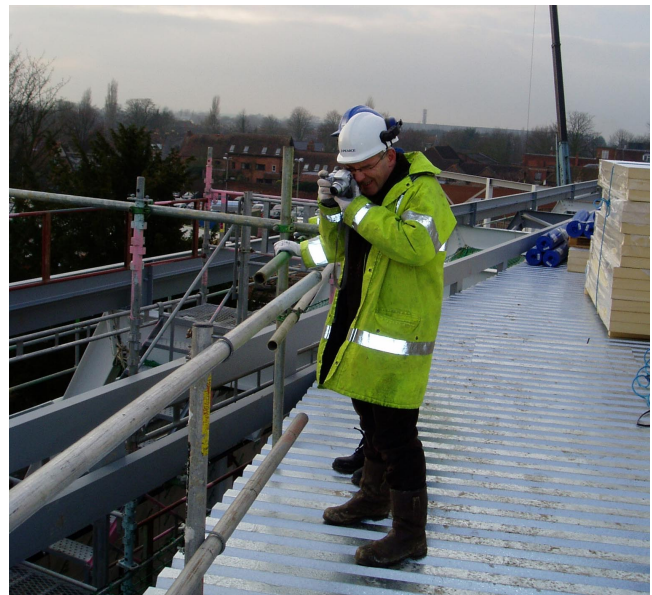
Figure 3. Health and safety audit
