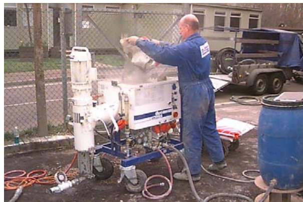
Figure 3. Dual-mixing wet-process pump in operation
