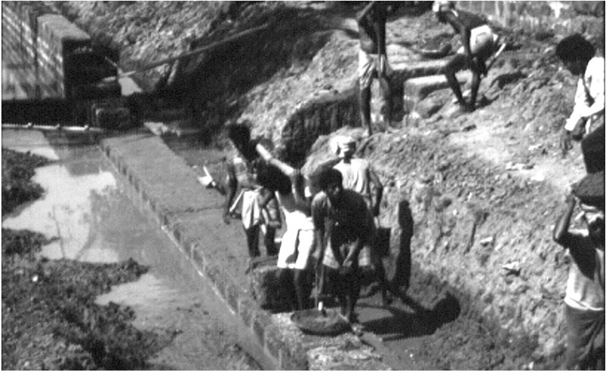
Photograph 2: Micro contractors improving secondary drainage, Cuttack, India
