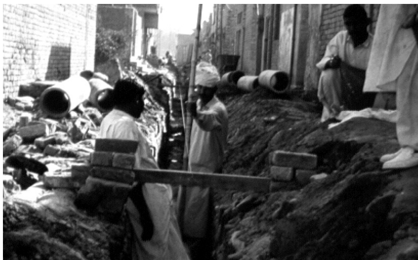
Photograph 6: Community management of sewer construction, Faisalabad, Pakistan
