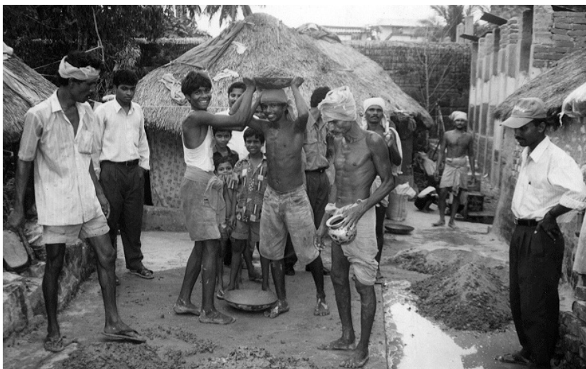
Photograph 4: Community contractors construct a concrete lane, Cuttack, India
