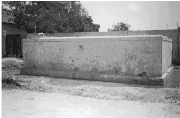
Photograph 5.4. View of a large tank in Ghaziabad. The taps were stolen, so now the water is distributed through pails, buckets, and rope.
