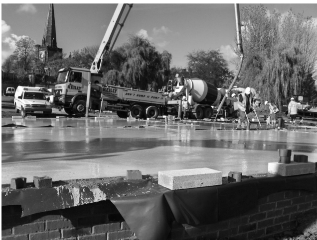
Figure 6. The most popular application of SCC was for slabs (courtesy of Lafarge)
