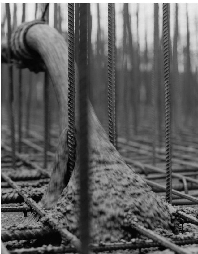
Figure 1. Self-compacting concrete in use (courtesy of Lafarge)
