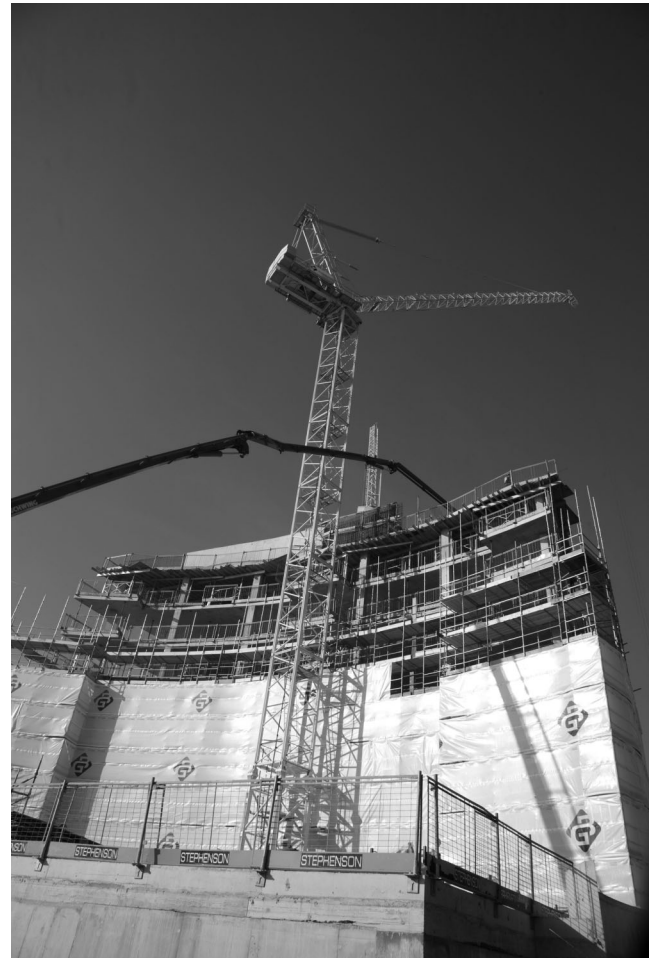
Figure 2. First major UK concrete frame constructed with SCC (courtesy of Lafarge)
