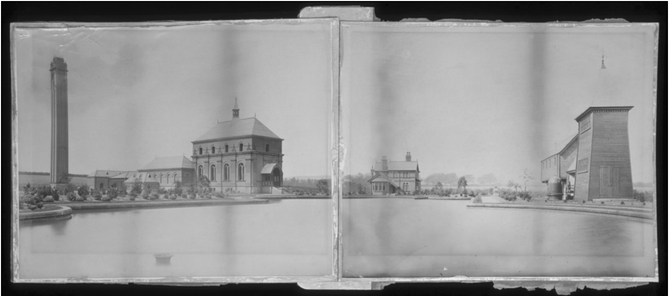
Fig. 4. Papplewick Pumping Station 1886 (Papplewick Pumping Station Museum, Notts)
