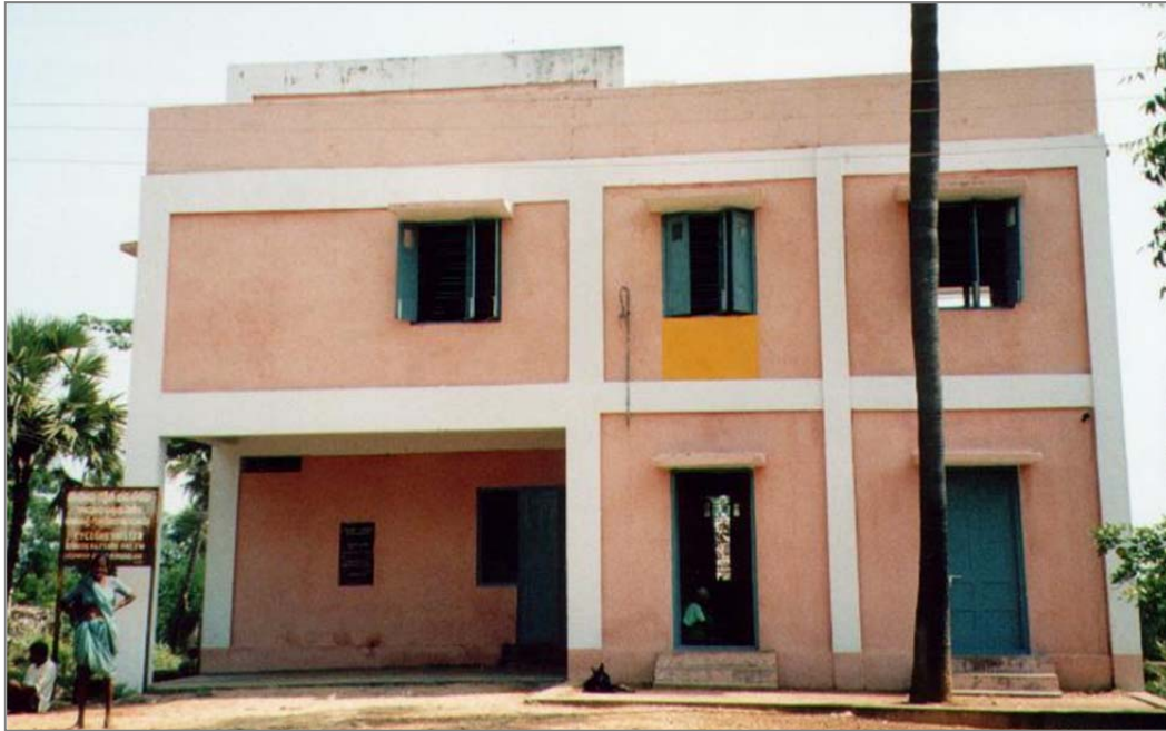
Photograph 5.2: Kottapattapalem Cyclone Shelter
