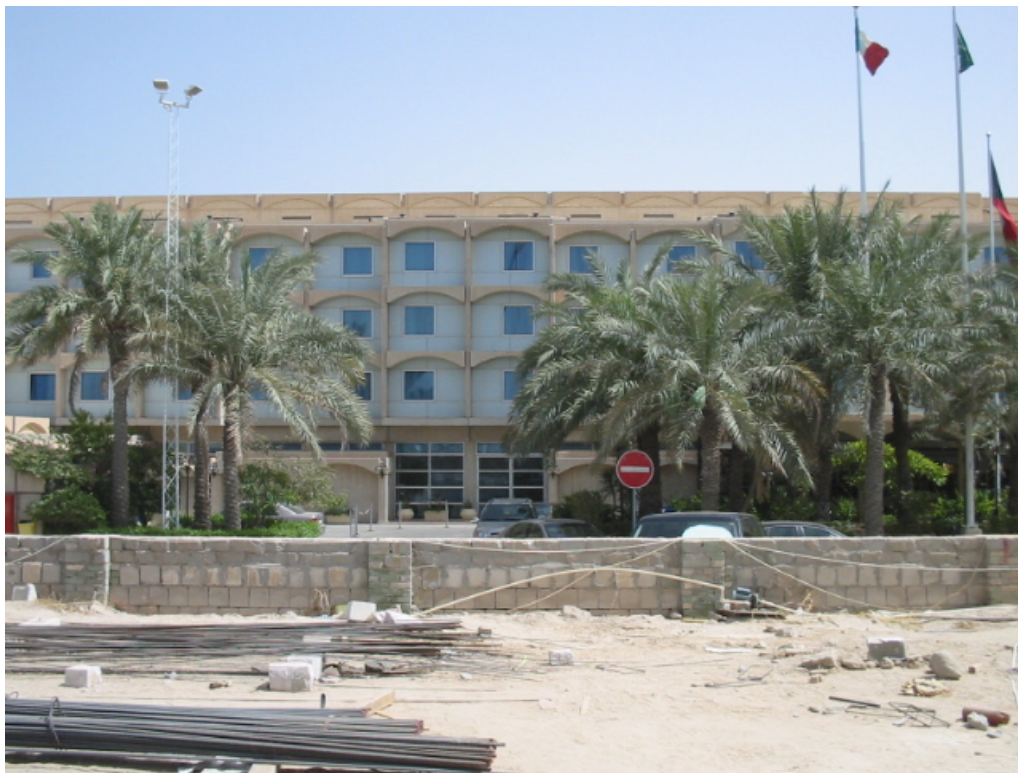
Fig. 3.50: A Hotel has four floors and Half in violation with BR 1985
