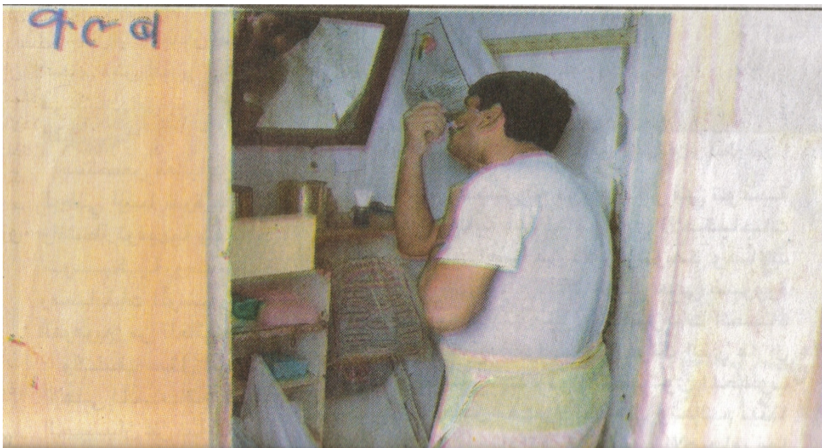
Fig. 3.36: Inappropriate toilet lacking many necessary health requirements
