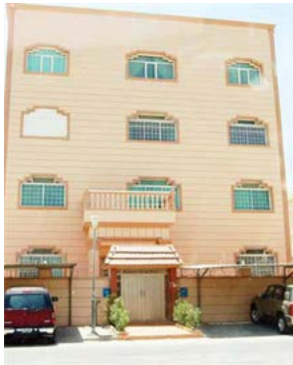
Fig. 3.54: A House (in Salwa) has four floors in violation with BR 1985
