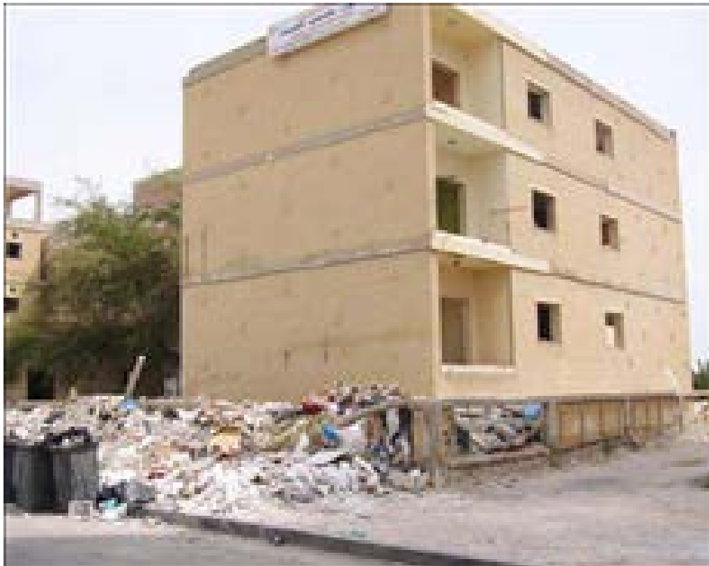
Fig. 3.28: Construction debris and wastes
