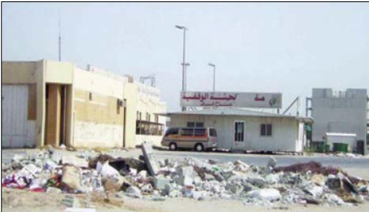
Fig. 3.25: Construction debris and wastes
