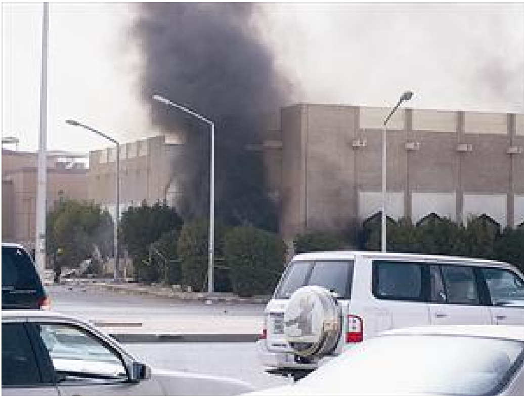
Fig. 3.42: Fire of merrymaking building in April 2009
