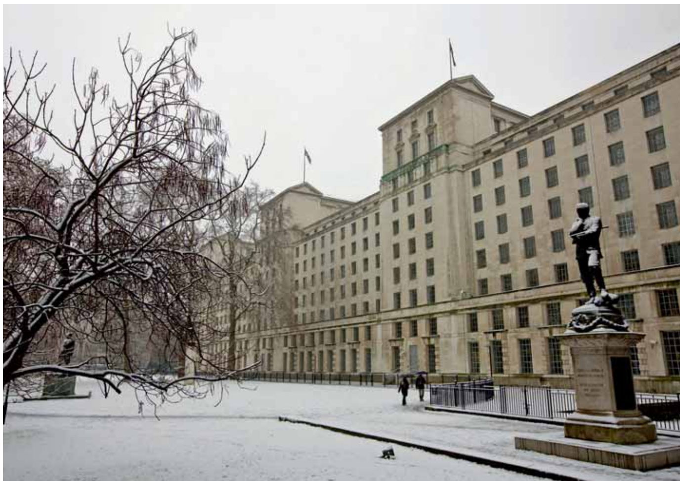
The MoD's Main Building in Whitehall, part of the Ministry's extensive property portfolio
