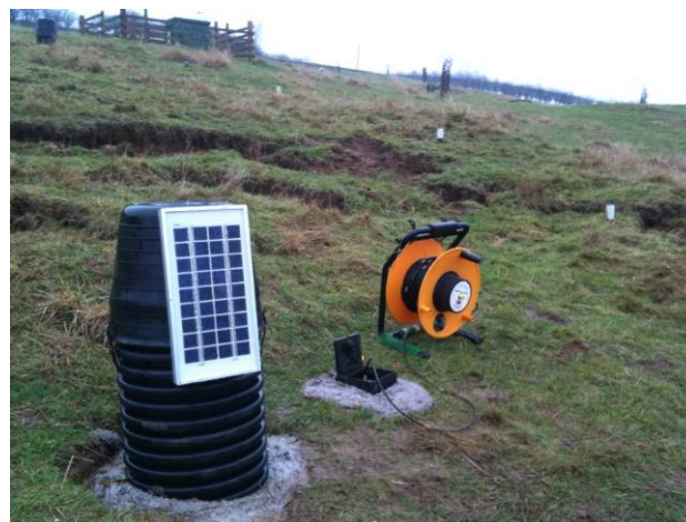
Figure 4. Acoustic waveguide with protective cover and adjacent inclinometer casing
