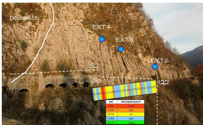
Figure 4. Projected RQD analysis from the S1 core on the west rock mass face, location of external extensometers and indicative location of inclinometer casing, waveguides and TDR cables.
