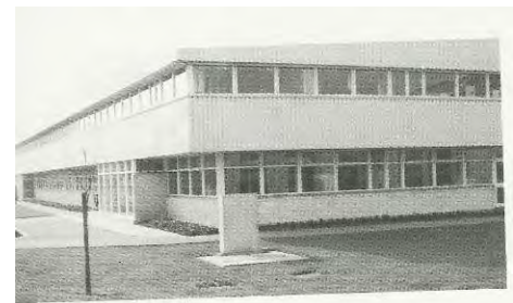
Fig.7.3 The 1960 purpose built workshops and the home of the Department of Design and Technology: the Bridgeman Centre
