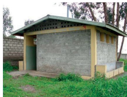
Figure 4. Latrine block with ramp access to entrance on left
