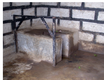
Figure 6. Raised toilet seat with support rail fixed to floor
