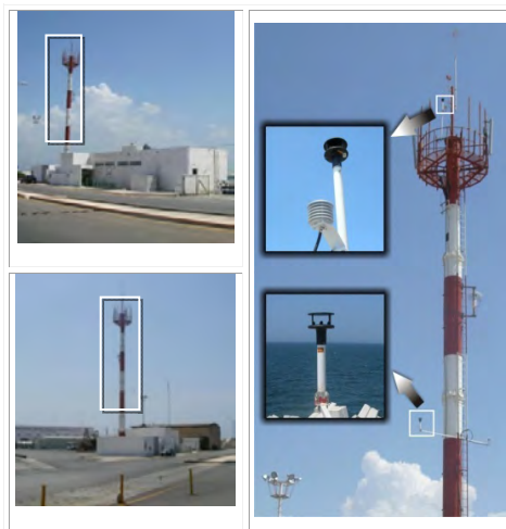
Figure 2. Different terrestrial views of the measurement tower showing the location of the tower on the pier and the position of the sensors on the tower.
