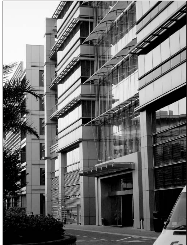
Fig. 2. Solar shading is essential but often woefully inadequate in highly glazed modern buildings
