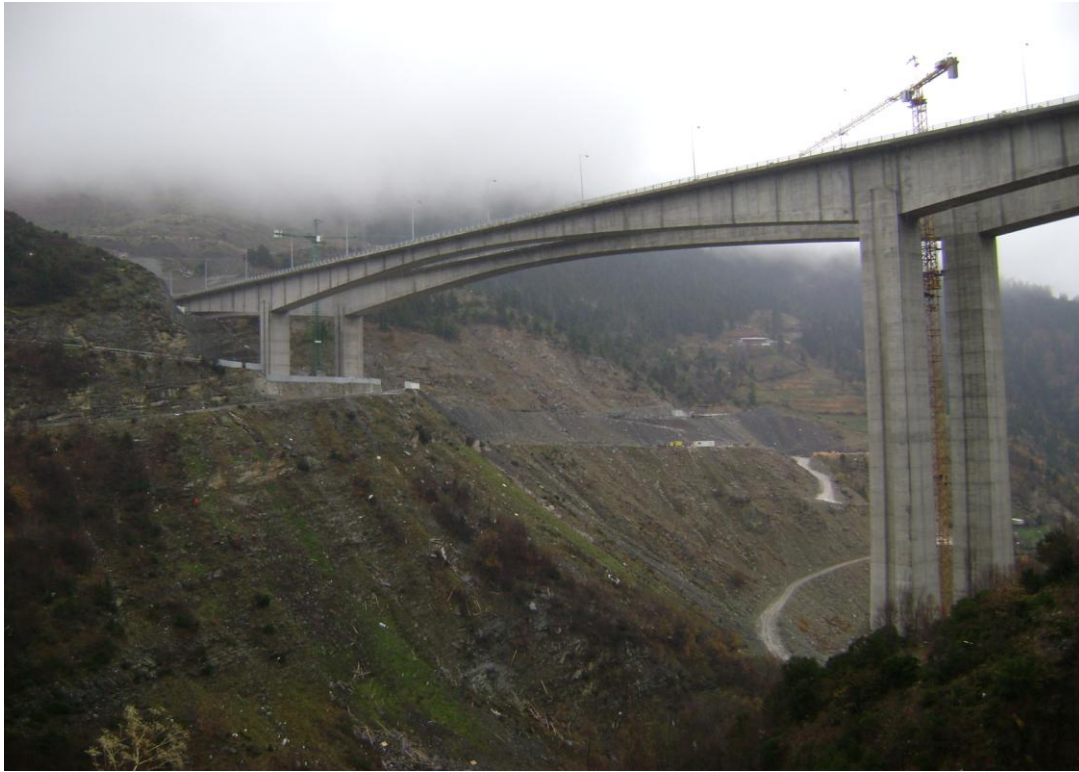
Figure 1: General view of Metsovo ravine bridge.
